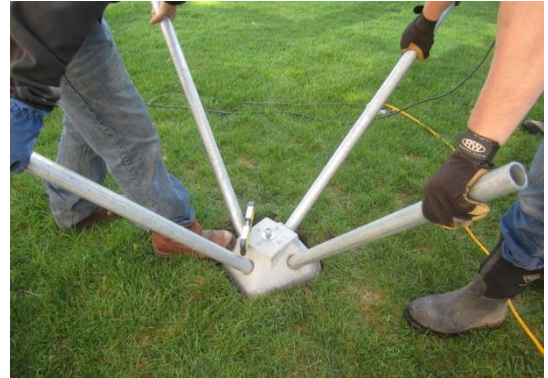
Figure 6. Setting Pins and Leveling Concrete Head
