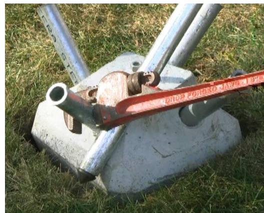
Figure 8. Jacking Method for Pin Removal
