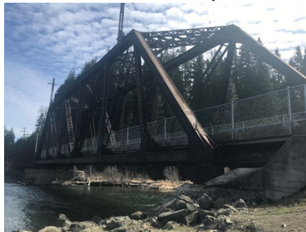
Palouse to Cascades Trail – FF-2 (Yakima River Bridge) - 1-150' thru truss, 1-150' thru plate; 303' length. This is a Non-Reportable Pedestrian structure used by Parks maintenance, contractors, and non-Parks utility maintenance vehicles.
