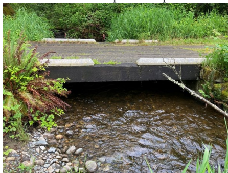
Lake Sammamish State Park – Group Camp Bridge - Timber 18" wide by 12" high timber beams on concrete footings, plastic curb stops used as side rails. This is a Non-Reportable Vehicular structure and is open to the public.
