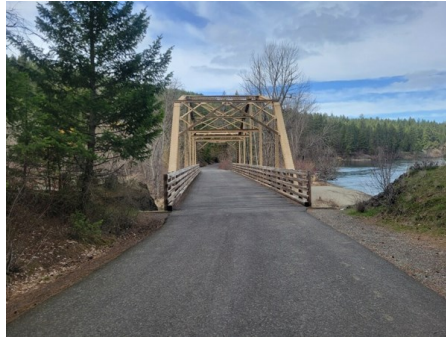
Palouse to Cascades Trail – FF-2 (Yakima River Bridge) - 1-150' thru truss, 1-150' thru plate; 303' length. This is a Non-Reportable Pedestrian structure used by Parks maintenance, contractors, and non-Parks utility maintenance vehicles.
